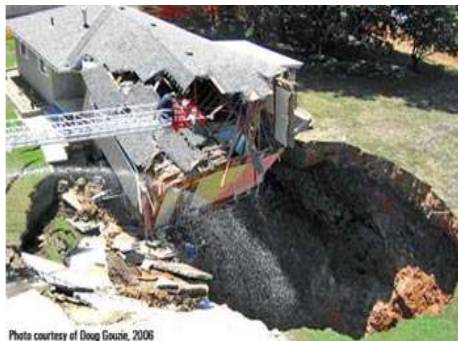
Figure D-11. Sinkhole Collapse of House
