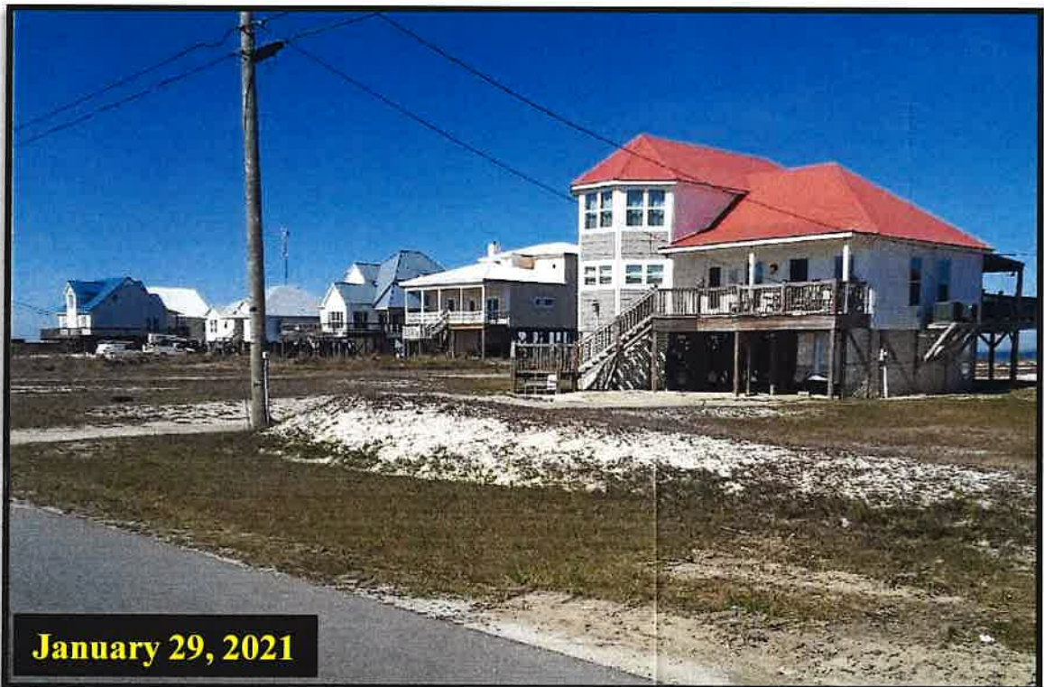
Photo 4. View of small sand berm on north side of Bienville Blvd.
