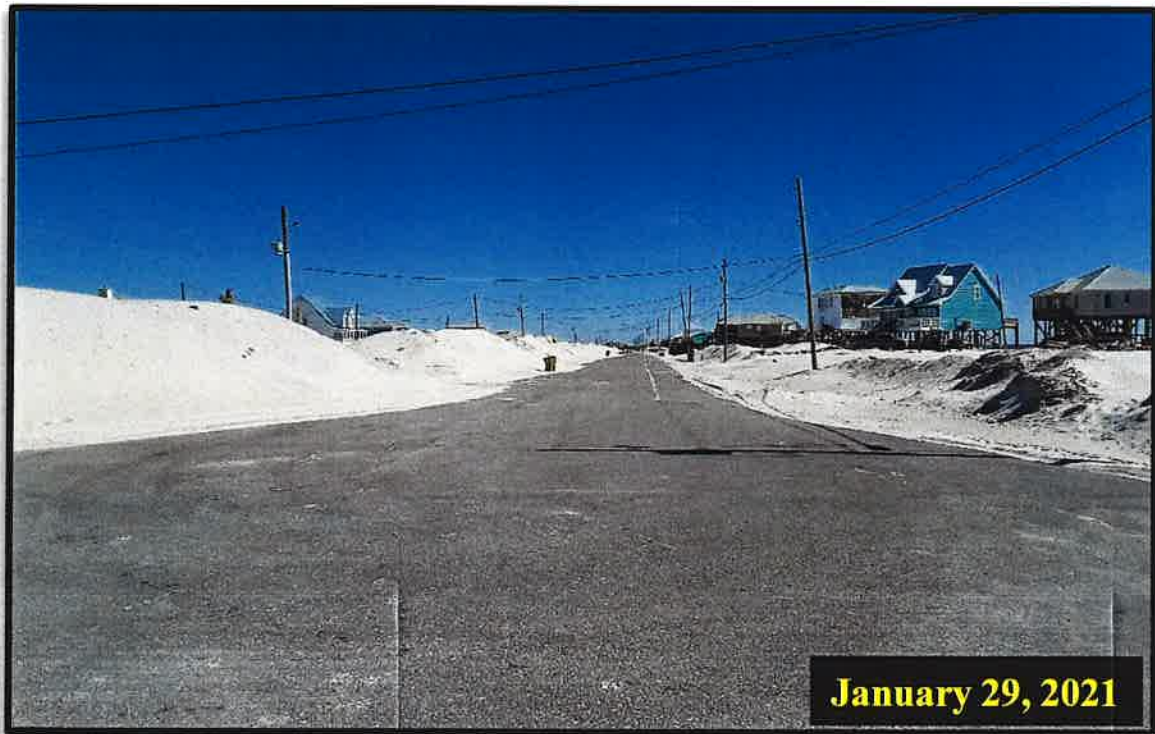
Photo 10. View looking east down Bienville Blvd showing piled sand on sides of road
