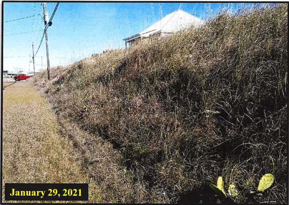
Photo 5. View of densely vegetated berm on south side of Bienville Blvd
