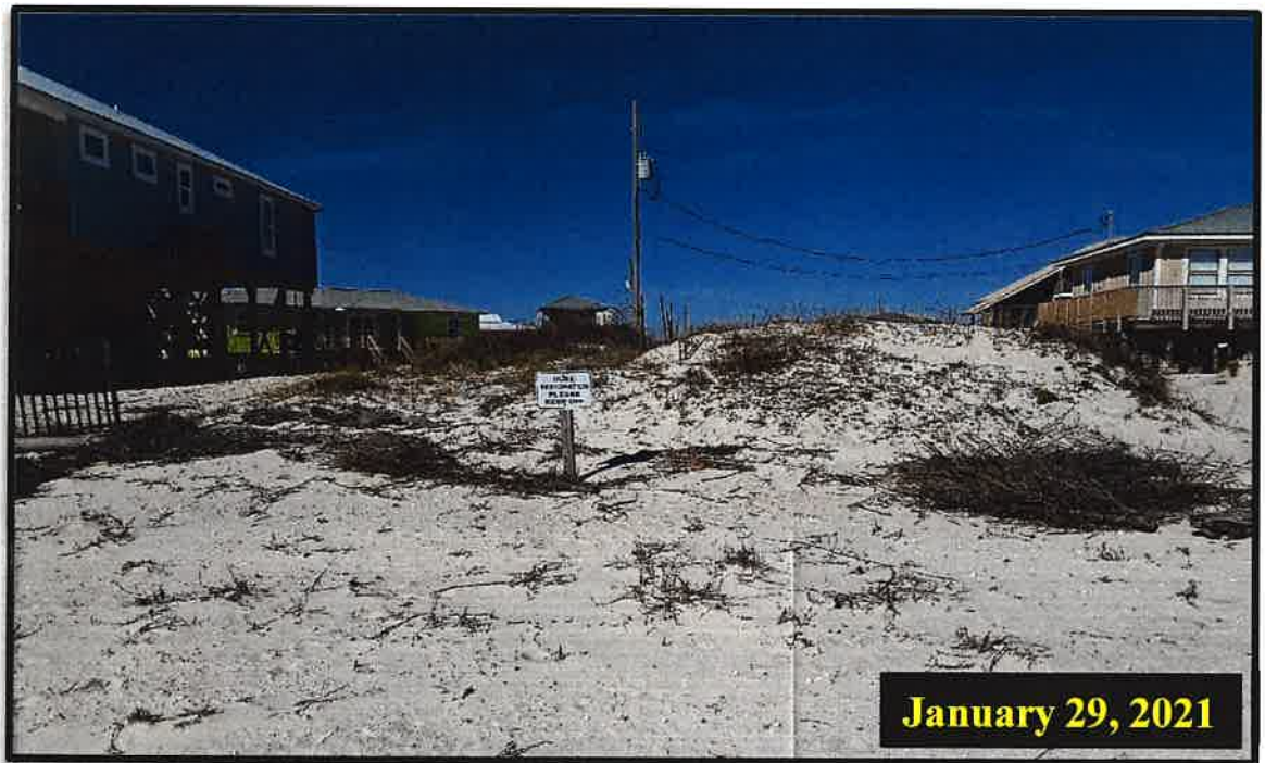
Photo 8. View of dune restoration on Ponce de Leon Court
